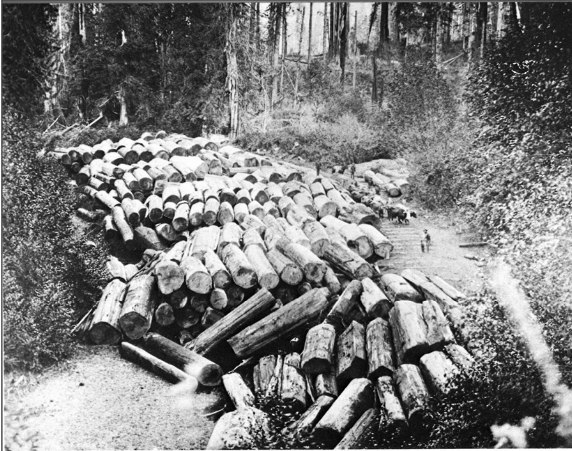
Figure 6-1. Logs stacked in Elk River in 1892, waiting for a winter freshet to carry them downstream. Seth Buck Collection.
