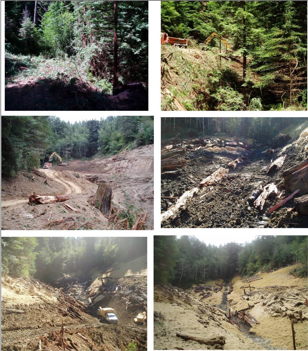
Figure 4-22. Time sequenced photographs of the excavation of the “Big Dig” site.
