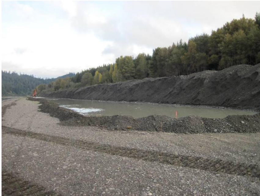
Figure 5. Excavator and trench on Truck Shop Bar during 2012 operations (2014 operations similar).
