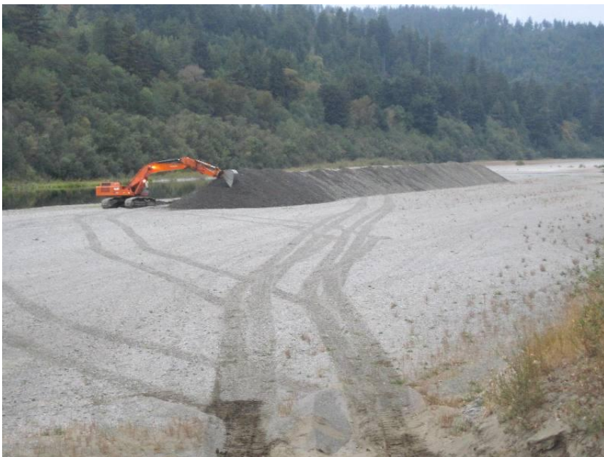
Figure 4. Excavator on Truck Shop Bar during 2012 operations (2014 operations similar).
