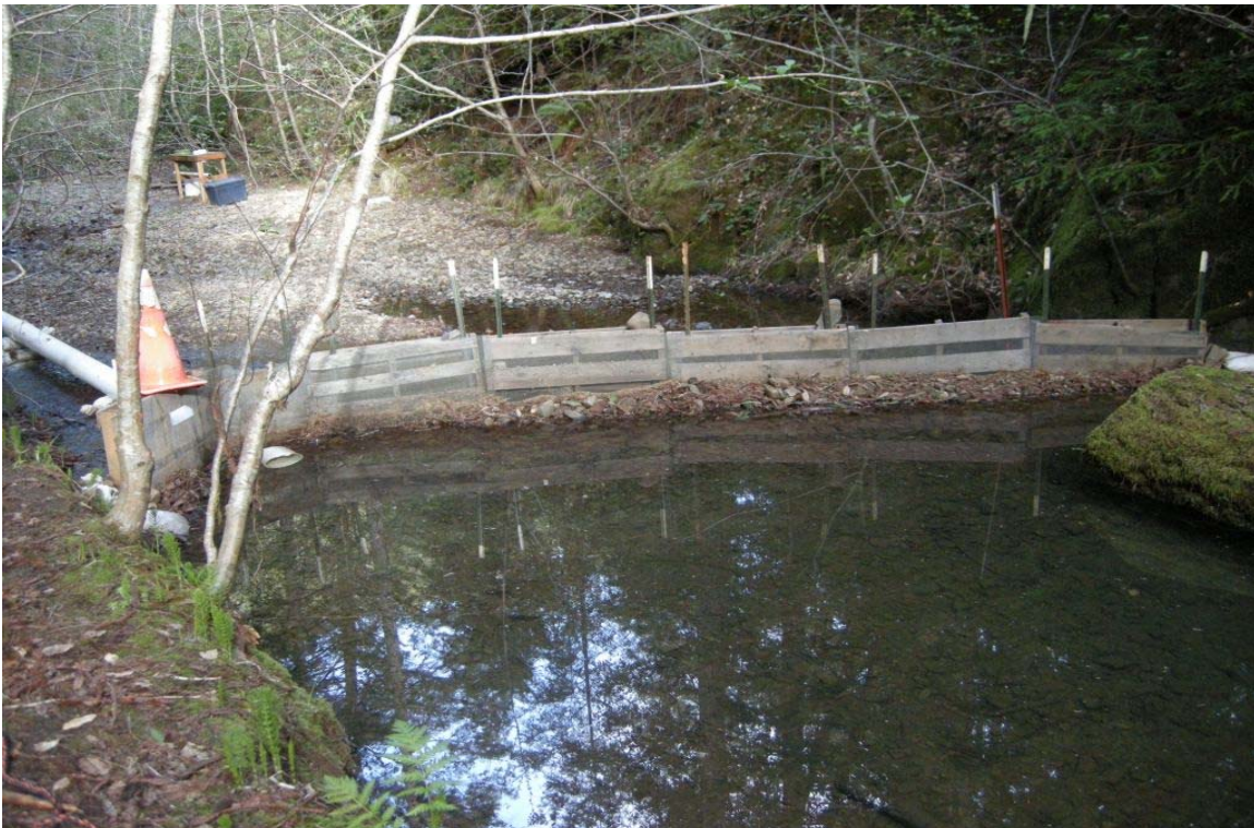
Figure 1. A pipe trap weir located in the Little North Fork Navarro River 2009.
