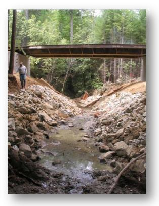
In July 2010, the MRC Road Department crew worked to complete the restoration project. They removed the sediment (dirt) surrounding the culvert to a safe location, removed the culvert itself, re-aligned the gradient of the stream to allow for fish passage, and placed the bridge to safely cross the new stream channel.
