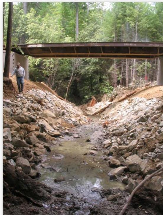
In July 2010, the MRC Road Department crew worked to complete the restoration project. They removed the sediment (dirt) surrounding the culvert to a safe location, removed the culvert itself, re-aligned the gradient of the stream to allow for fish passage, and placed the bridge to safely cross the new stream channel.
