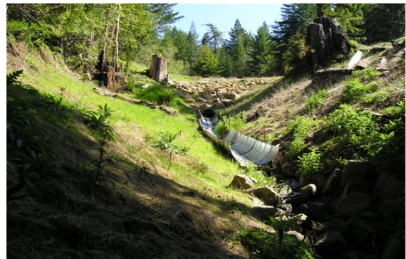
Stormproofed Stream Crossing – Elk River Watershed
