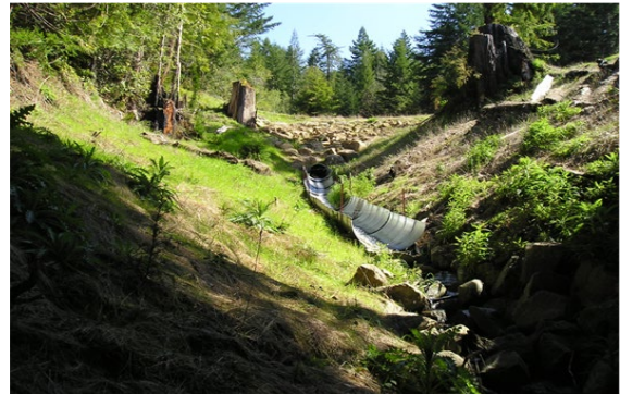
Stormproofed Stream Crossing – Elk River Watershed
