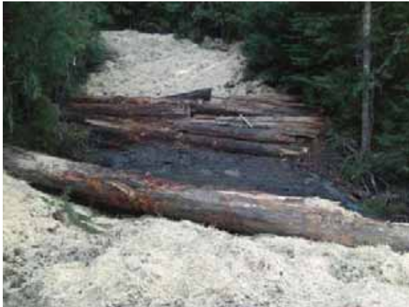
Same site on January 19, 2009 after pulling the wood and soil out of the stream – note the straw mulch placed on disturbed soil
