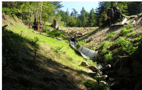
Stormproofed Stream Crossing – Elk River Watershed
