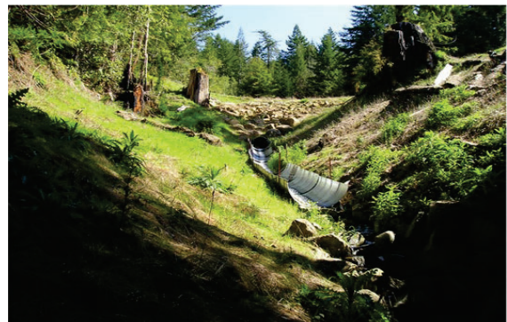
Stormproofed Stream Crossing – Elk River Watershed
